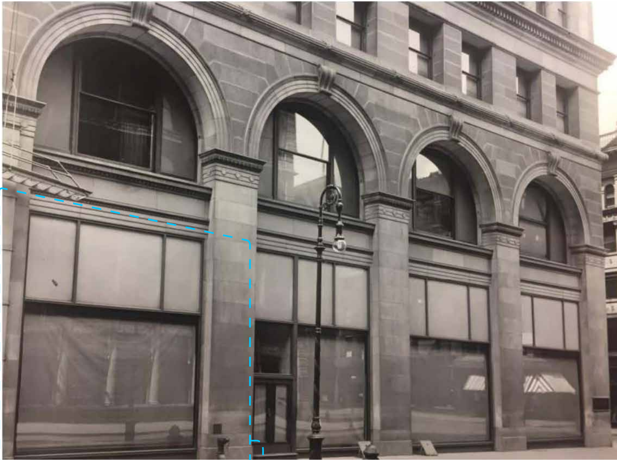
1 | NW Corner Broadway & 9th Street Looking SW (1913) └─ New Entry Bay in Scope of Work
